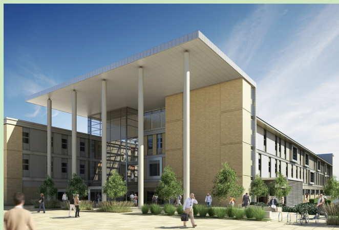
If you haven't seen the new South Bristol Community Hospital (pictured) yet, please get in touch to arrange a visit
